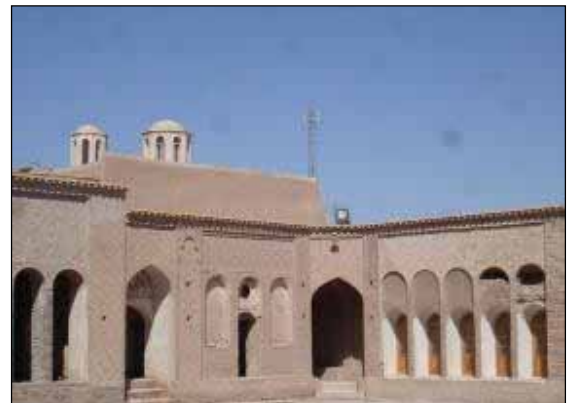
Figure 12. Southern Iwan (porch)
