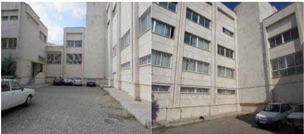
Figure 7. The windward and blast wave intensifier angles in the plan for the central library of Tabriz
