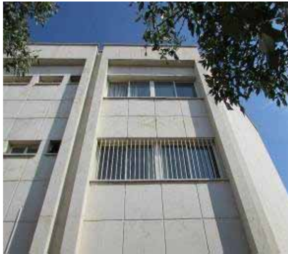
Figure 8. The bleach in the height of the building of the central library of Tabriz
