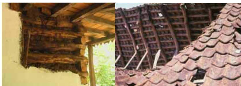
Figure 4 & 5. Construction detail of interlocking log wall and roof tiles (Source: Author)
