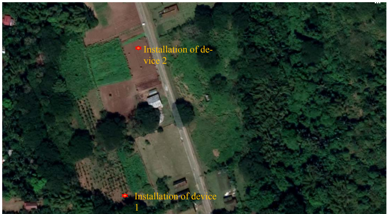
Figure 1. Site Location of SPSMMS installations
