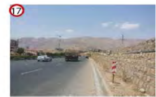
Figure 11: View of Hashemi Expressway
