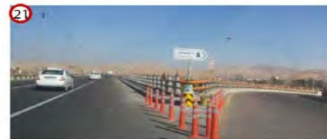
Figure 14: View of Hashemi Expressway
