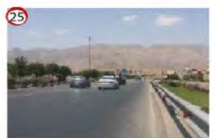
Figure 13: View of Hashemi Expressway
