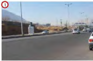
Figure 3:View of Hashemi Expressway
