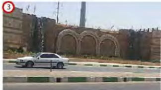
Figure 5:View of Hashemi Expressway
