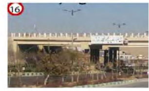
Figure 10: View of Hashemi Expressway
