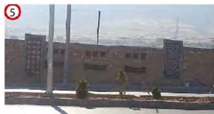
Figure 7:View of Hashemi Expressway
