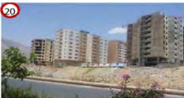
Figure 15: View of Hashemi Expressway
