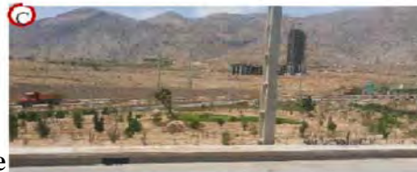
Figure 12: View of Hashemi Expressway
