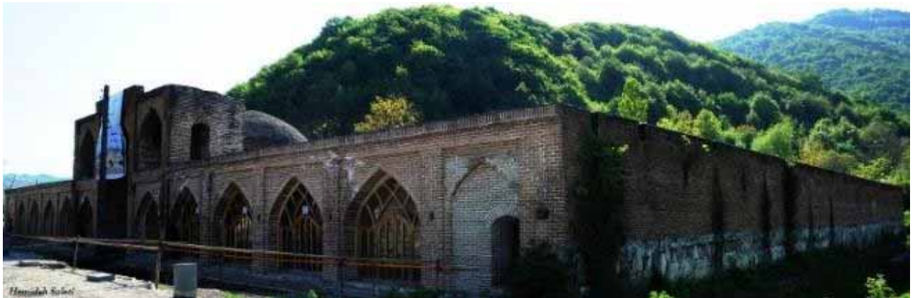
Figure 13: Rasht, Lat Caravanserai
