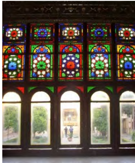
Figure 4. Sash windows in the house of Zinatolmolk, Qajar era, Shiraz, upside of windows is knurled with colorful glasses and ceiling is decorated with mirror (Source: Author)
