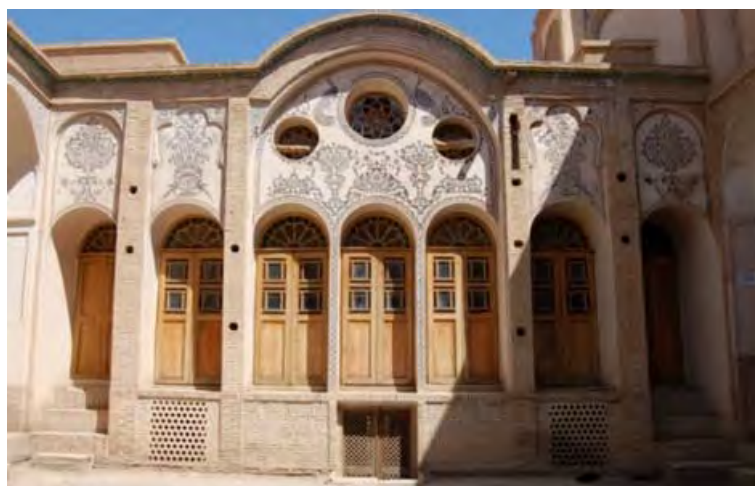
Figure 5: Outside of five-door room of Borojerdiha house, Kashan, Two doors in the right and left belong to the corridor and each window has two doors (Source: Author)
