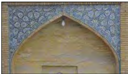
Figure 9. gere accomplished in the western-side spandrel
