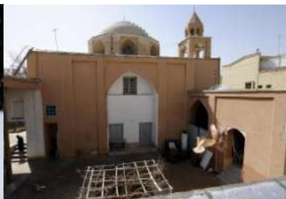
Figure 8. St. Nicholas church (exterior view)
