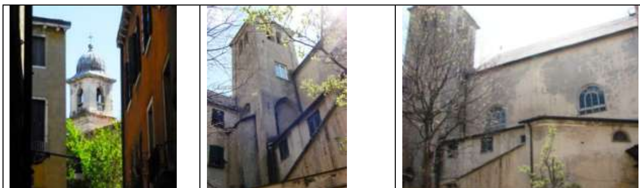
Figure 7. Remains of the ancient church, including the bell tower
