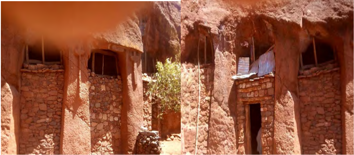
Figure 2. External columns visible and missing crosses Photo source: by researcher (March 24, 2020)
