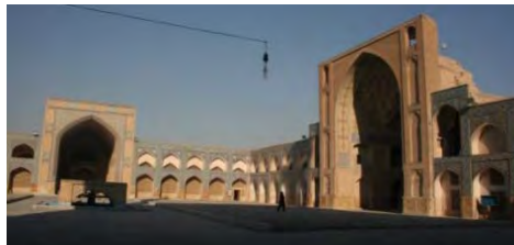
Image 1. The west veranda (right) and south veranda(left) of Isfahan Jame(Atiq)Mosque (Authors, 2014)
