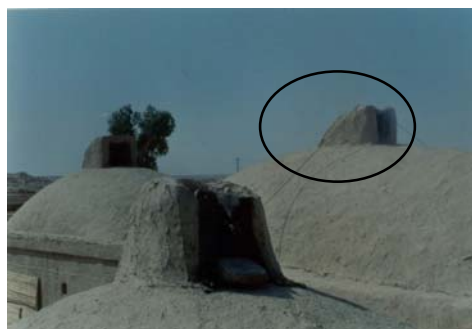
Figure 4: Sistan region wind tower (Source: author)
