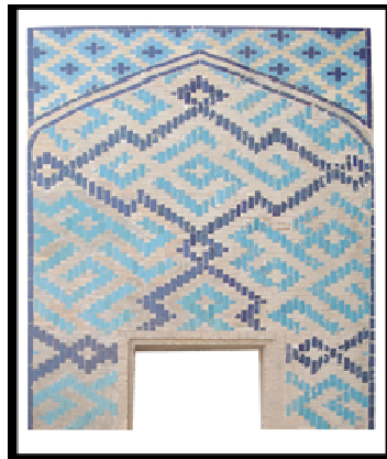
Fig 12: Part of southern façade
