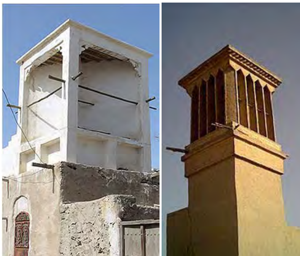
Figure 15: White windcatchers of Loft harbor (left) Yazd windcatchers (right)
