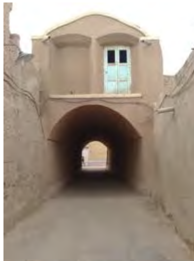
Figure 6. An archway with a room on top
