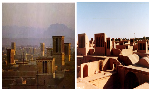
Figure 14. One-way windcatchers in Ardakan (right) and four sided windcatchers at Yazd (left)
