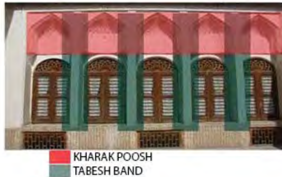
Figure 3. The location of vault and light hedge on building facade
