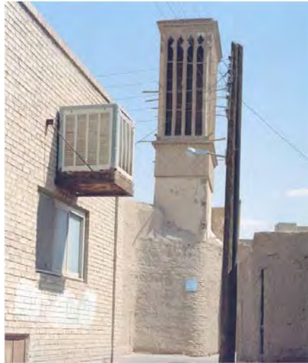
Figure 16. Comparison of historical and contemporary home cooling facilities
